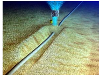
Post Lay Trenching
